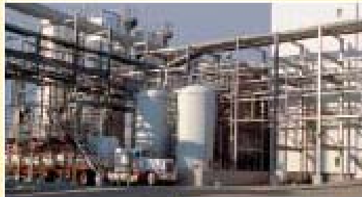
Left and below: Harbor Beach spinosad fermentation facility
