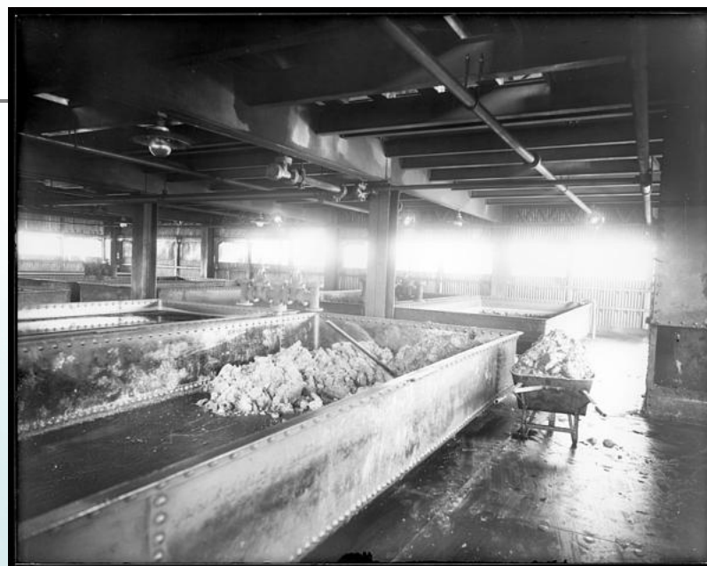
Coke Plant Naphthalene Settling Pans, 1916
